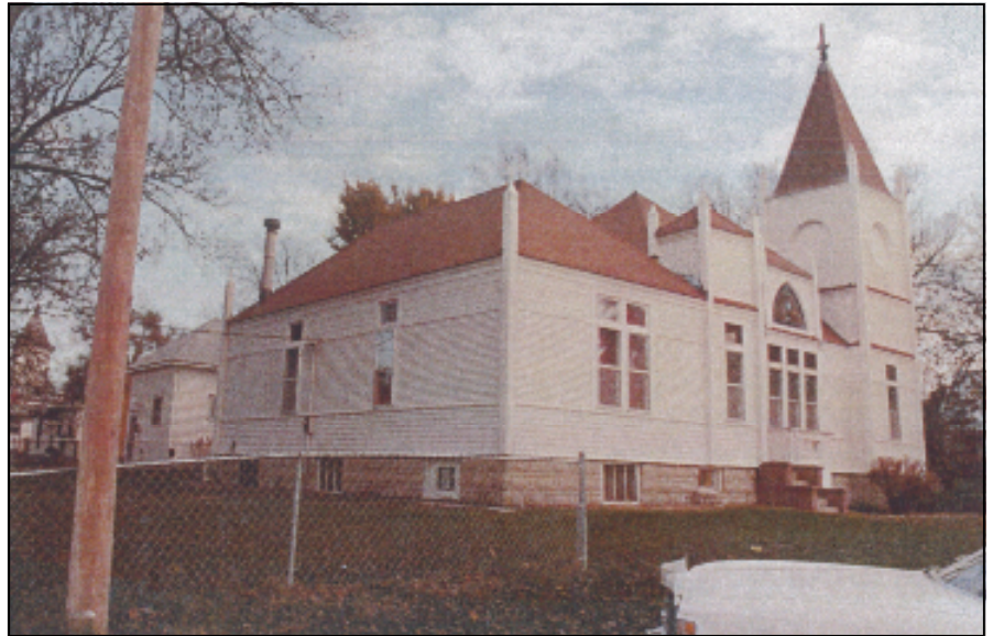
Original church building on North 10th Avenue
